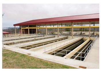
DE NORA TETRA<sup>TM</sup> DeepBed<sup>TM</sup> filters can easily meet <2 NTU or <5 mg/L TSS (<2 mg/L typical). Due to the filter's high loading capacity, the percent of dirty backwash water return is less than 4% (<2% typical) of the plant's forward flow.
