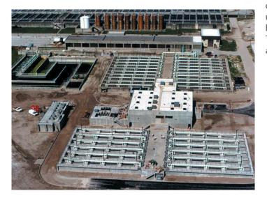
Denite<sup>®</sup> is a fixed-film biological denitrification process that also serves as a deep bed filtration system capable of removing suspended solids to a level of 2-3 mg/L. Denite<sup>®</sup> can be used as part of a process to help facilities meet stringent TN discharge limits as low as 3 mg/L.
